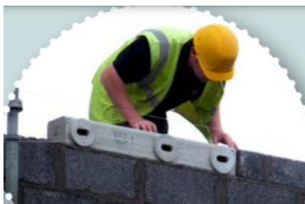
Integrating a Swift nest box into a building
